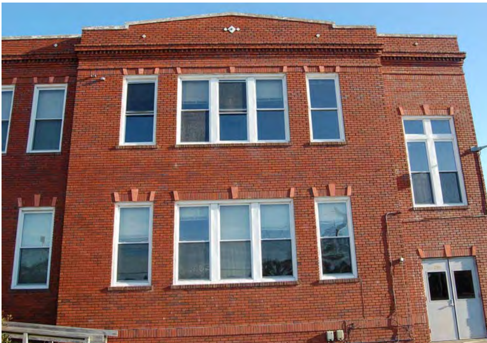
Plate 52. Topsail Consolidated School, Façade, South Classroom Bay, Looking Southeast.
