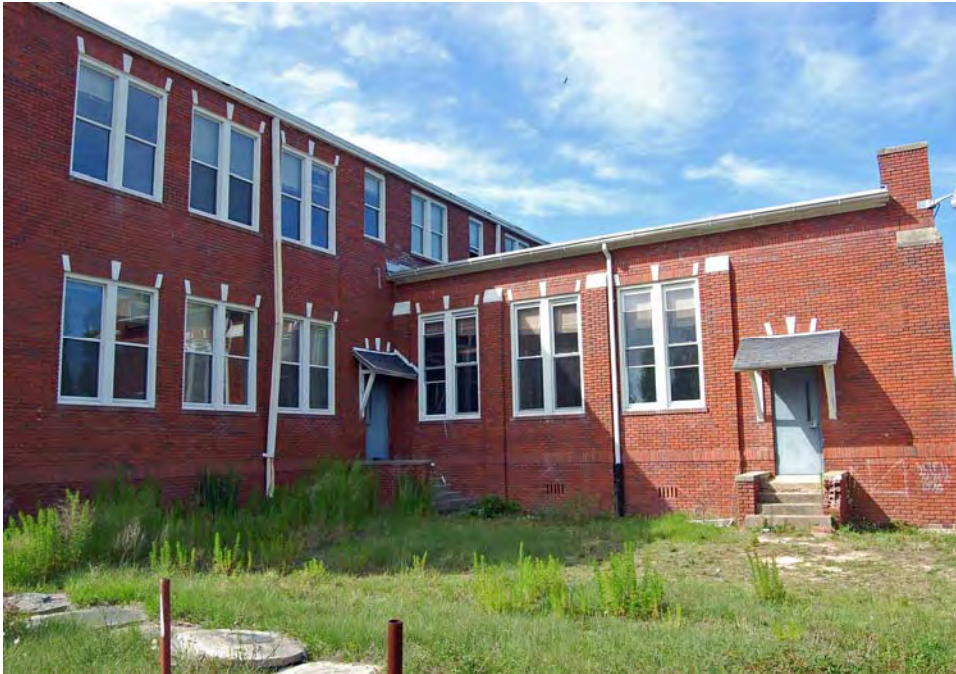
Plate 55. Topsail Consolidated School, Rear Elevation and Rear Auditorium Wing, Looking North.
