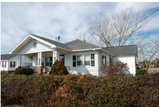
No. 37 House (PIN 3282-00-9177-0000) 10 Browntown Road, Scotts Hill
