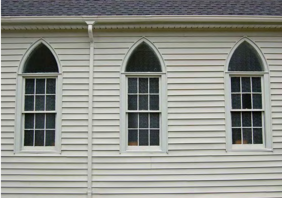
Plate 15. Mount Ararat AME Church, South Elevation, Windows, Looking North.
