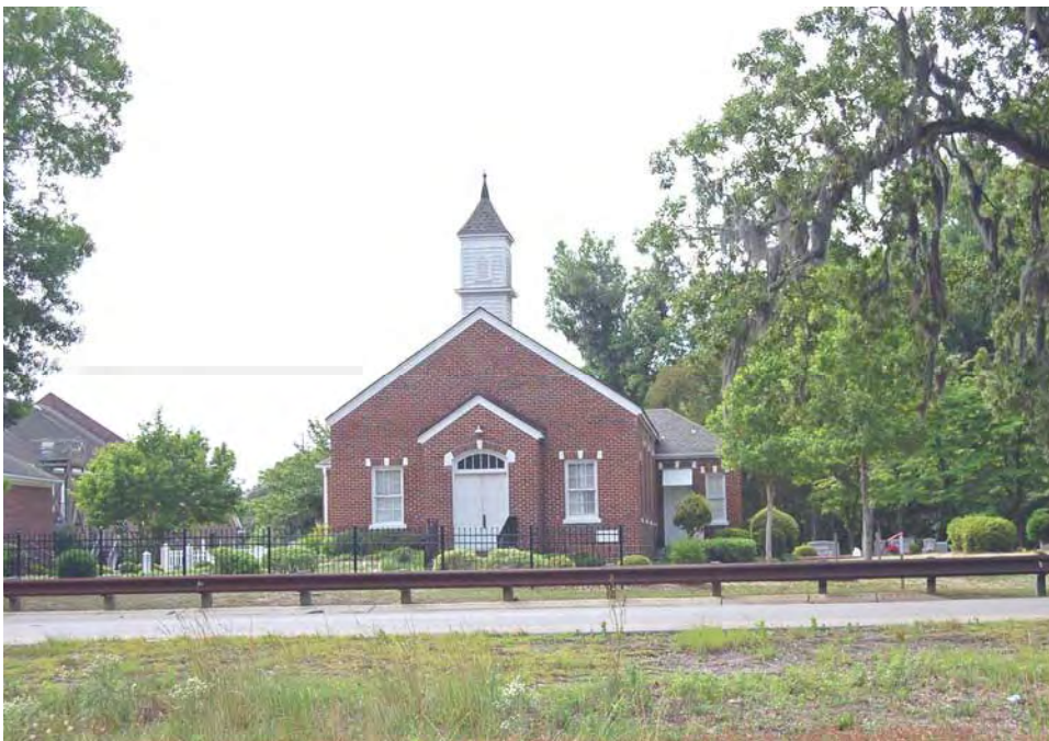
Plate 28. Wesleyan Chapel United Methodist Church, 1931 Church, Looking West Across US 17.
