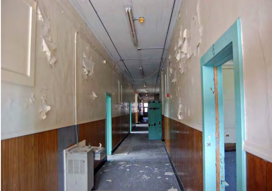
Plate 59. Topsail Consolidated School, Interior, First Floor Corridor, Looking North.
