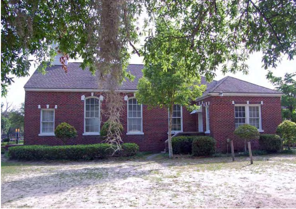
Plate 33. Wesleyan Chapel United Methodist Church, 1931 Church, Side (North) Elevation, Looking South.
