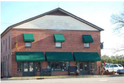
No. 44 Store (PIN 3282-97-1166-0000) 14712-14714 US 17 North, Hampstead
