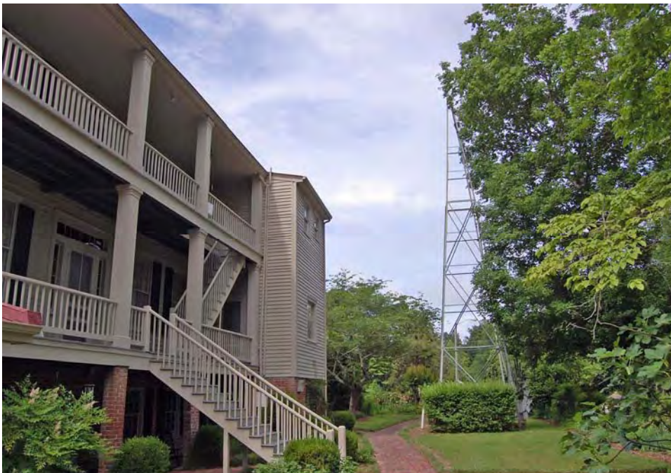
Plate 6. Poplar Grove, Rear (East) Elevation and Windmill, Looking North.
