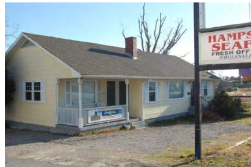
No. 45 Duplex (PIN 3282-97-6579-0000) 14820 US 17 North, Hampstead
