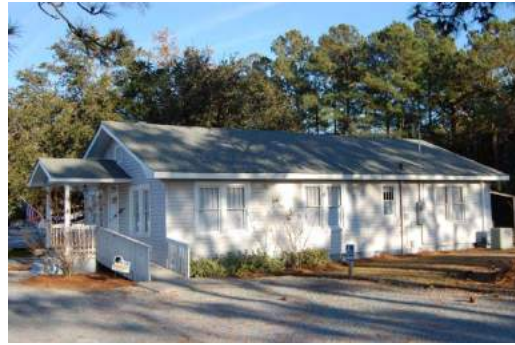
No. 78 House (PIN 4203-07-1431-000L) 17550 US 17 North, Topsail
