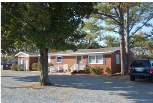
No. 5 House (PIN R05006-003-004-000) 6205 Market Street, Wilmington
