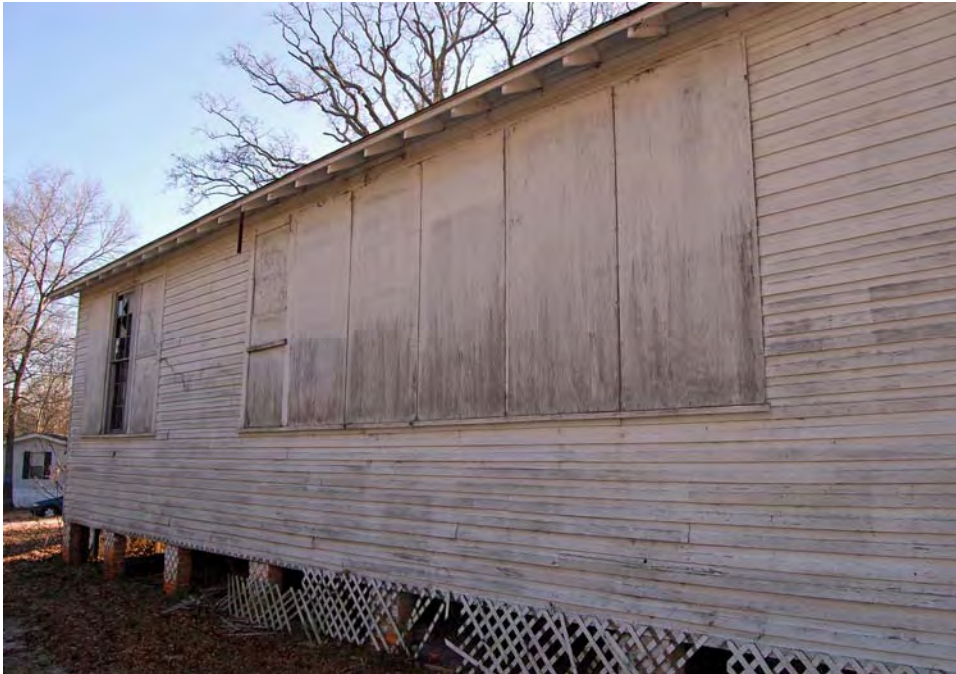
Plate 45. Scotts Hill Rosenwald School, Side (North) Elevation, Looking Southeast.
