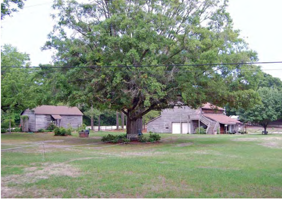
Plate 9. Poplar Grove, New Interpretative/Storage Buildings on the Site, Looking East.
