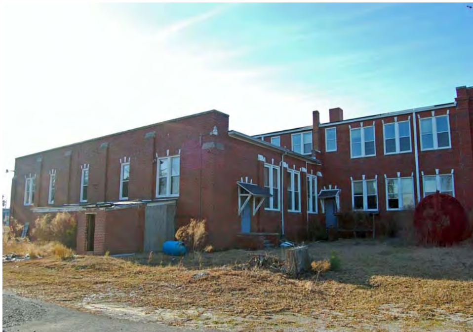
Plate 54. Topsail Consolidated School, Rear Elevation and Rear Auditorium Wing, Looking West.
