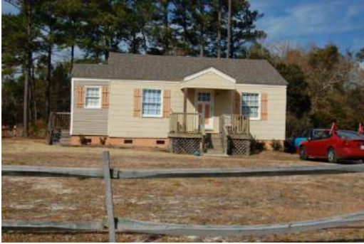
No. 33 House (PIN 3281-19-2053-0000) 164 Browntown Road, Scotts Hill
