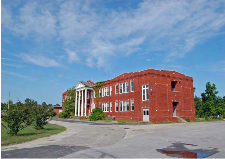
Plate 49. Topsail Consolidated School, School and Setting, Looking Northeast.
