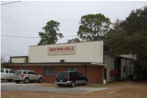
No. 3 Industrial Building (PIN R05009-005-027-000) 111 Old Eastwood Road, Wilmington
