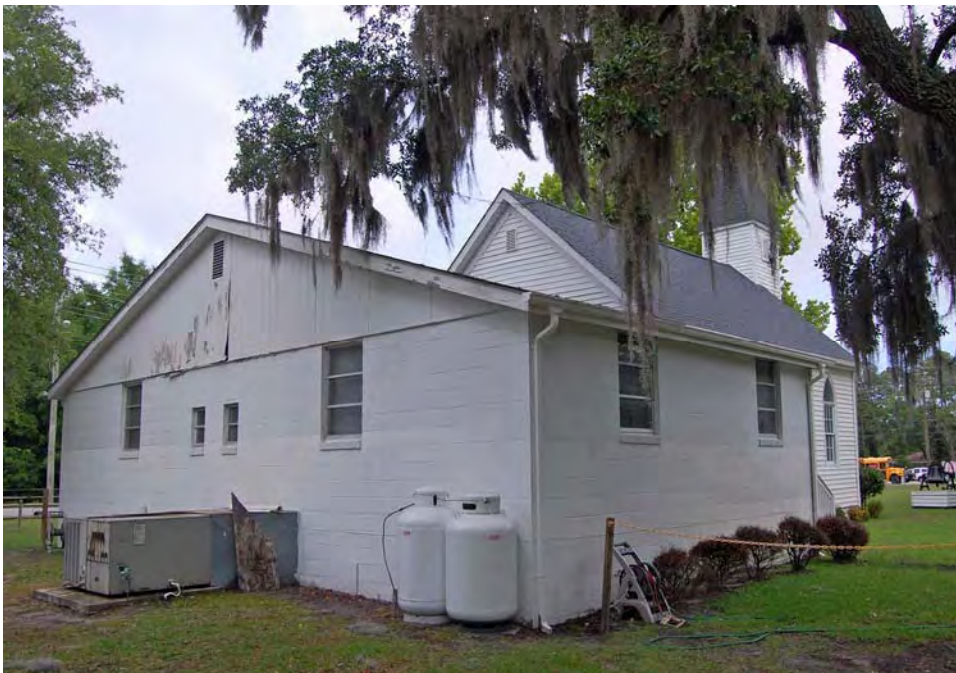
Plate 16. Mount Ararat AME Church, Rear Wing, Looking East.
