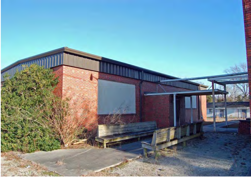
Plate 57. Topsail Consolidated School, Industrial Arts Building, Looking East.
