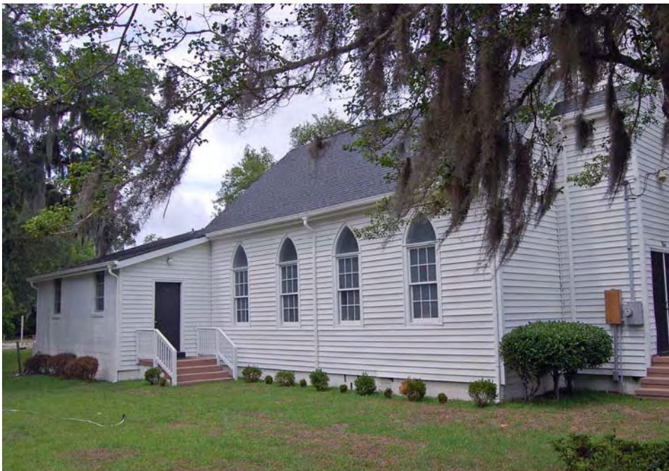
Plate 14. Mount Ararat AME Church, Side (South) Elevation, Looking Northwest.
