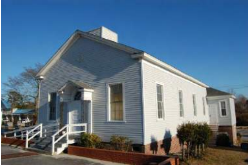
No. 46 Hampstead United Methodist Church (PIN 3282-97-6579-0000), 14840 US 17 North, Hampstead
