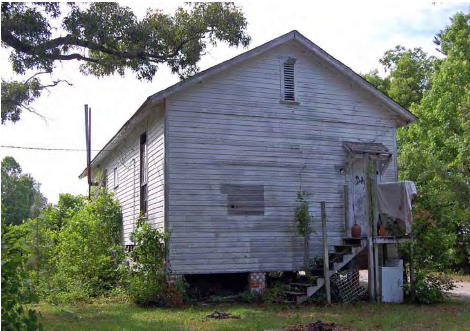
Plate 46. Scotts Hill Rosenwald School, Rear (East) Elevation, Looking West.
