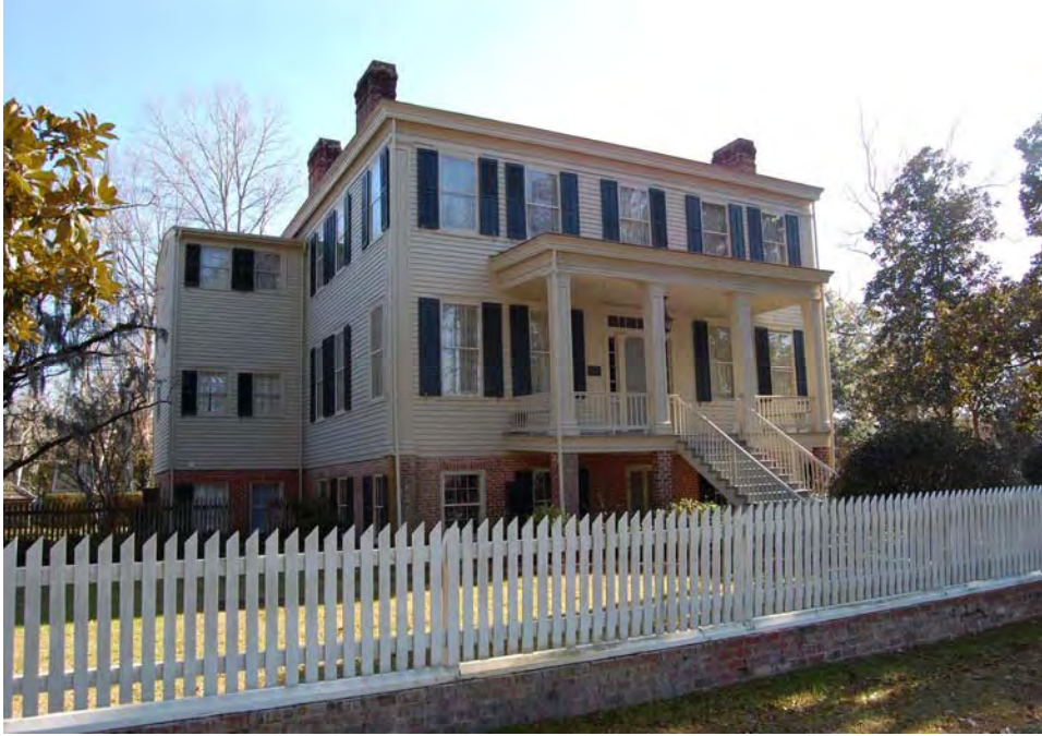
Plate 1. Poplar Grove, Façade, Looking East.
