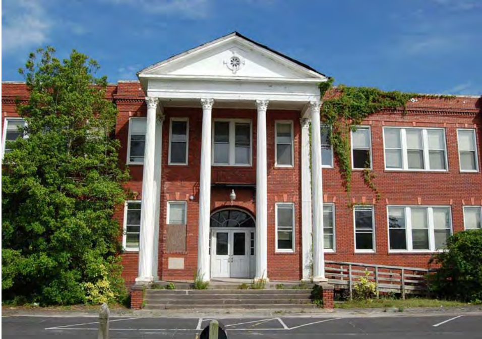
Plate 51. Topsail Consolidated School, Façade, Looking Southeast.
