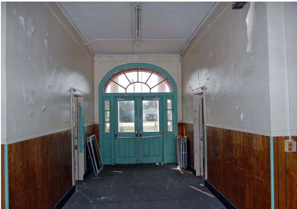
Plate 60. Topsail Consolidated School, Interior, Central Entrance Corridor, Looking West.
