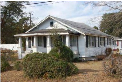
No. 35 House (PIN 3281-19-5342-0000) 34 Browntown Road, Scotts Hill
